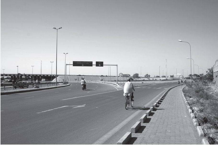
Figure 2.1 Southern Interchange, Ouagadougou (photograph: Jonas Haenggi).
