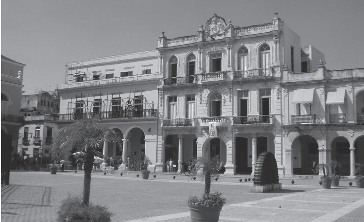
Fig. 7.3 Rehabilitation of the “Old Square” in Havana, Cuba, since 1979 (credit : A. Rabinovich).
