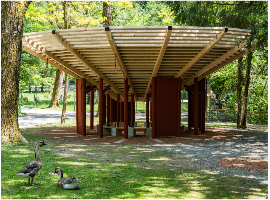
First build Form in 2019 by Students. Work in progress
