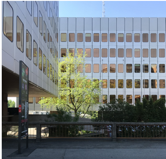
Atelier des Architectes Associés (AAA), Jean Prouvé, Chauderon Administrative Complex, Lausanne, 1970–1974 © Giulia Marino
