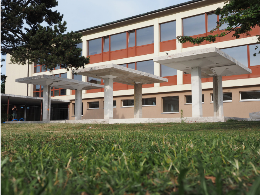
The design of the rebuiLT pavilion was deeply influenced by that of the reused saw-cut concrete assembly donor: an old mushroom-column and slab concrete structure. https://rebuilt.cargo.site © SXL, EPFL
